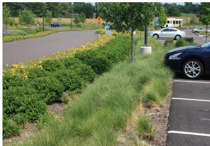
Infiltration trenches at Einstein Hospital in East Norriton.
