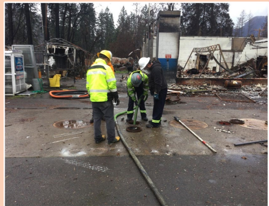
EPA contractors removing fuel from the USTs at Rivers Run Facility
