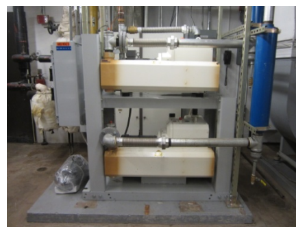
Anesthesia evacuation pumps
