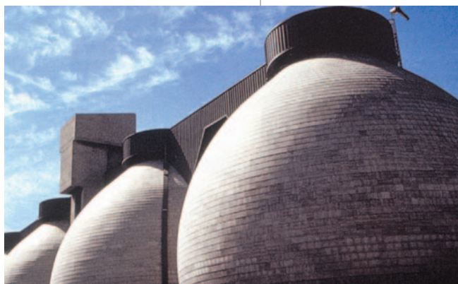
Egg-shaped Digestors
