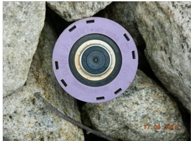
Figure 2-4 Purple snap-on reclaimed water identification cap (Photo credit: Rain Bird)
