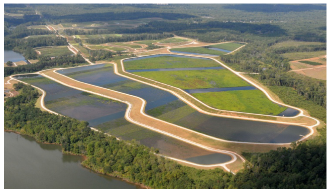
Figure 2 The E.L. Huie Constructed Wetlands (Photo credit: Aerial Innovations of Georgia, Inc.)
