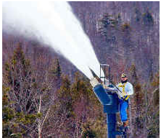
Figure 1 CVSD District employee Joseph Puleo checks the nozzles atop a snow gun tower. (Photo credit: David Keith)
