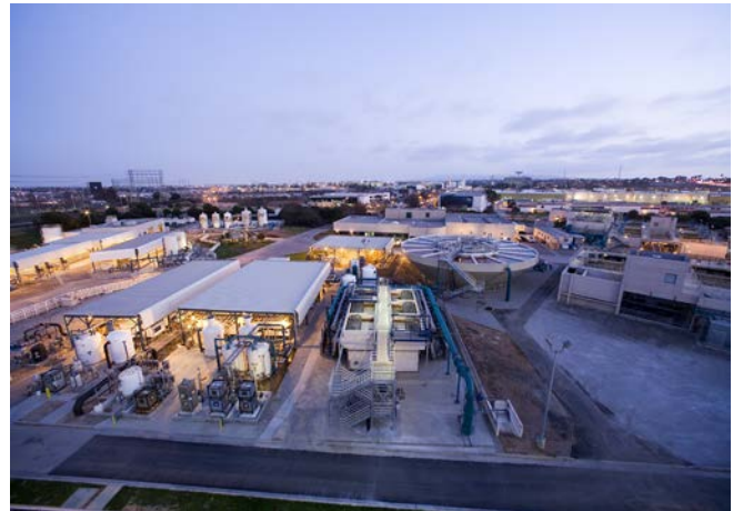
Figure 1 The Edward C. Little Water Recycling Facility is located in El Segundo, California
